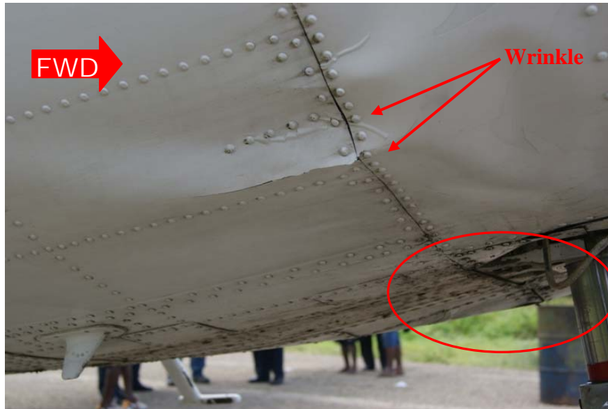
Figure 2. PK-NUH Station 60 (Lower Fuselage) Section
